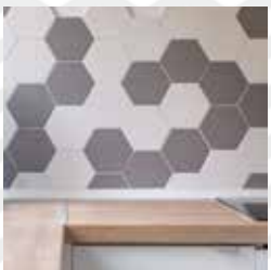
DADO CERAMIC TILES 600 MM ABOVE THE COUNTER
